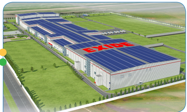
Exide Energy Solutions Limited, Bengaluru
