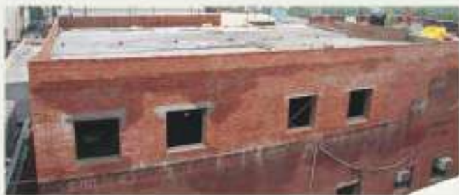
Exposed Brick Cladding
