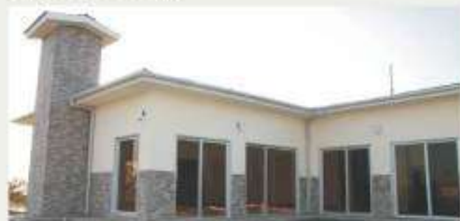
Wall Tile and Cement Board
