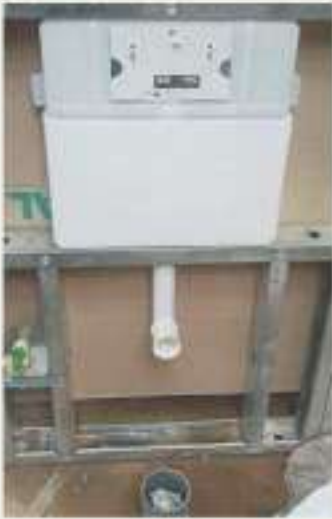
Wall / Floor mount WC Fixing Arrangement
