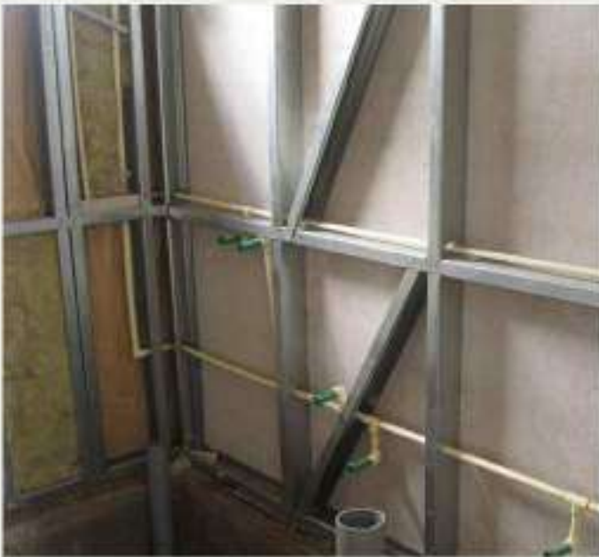
Geyser Fixing Arrangement
