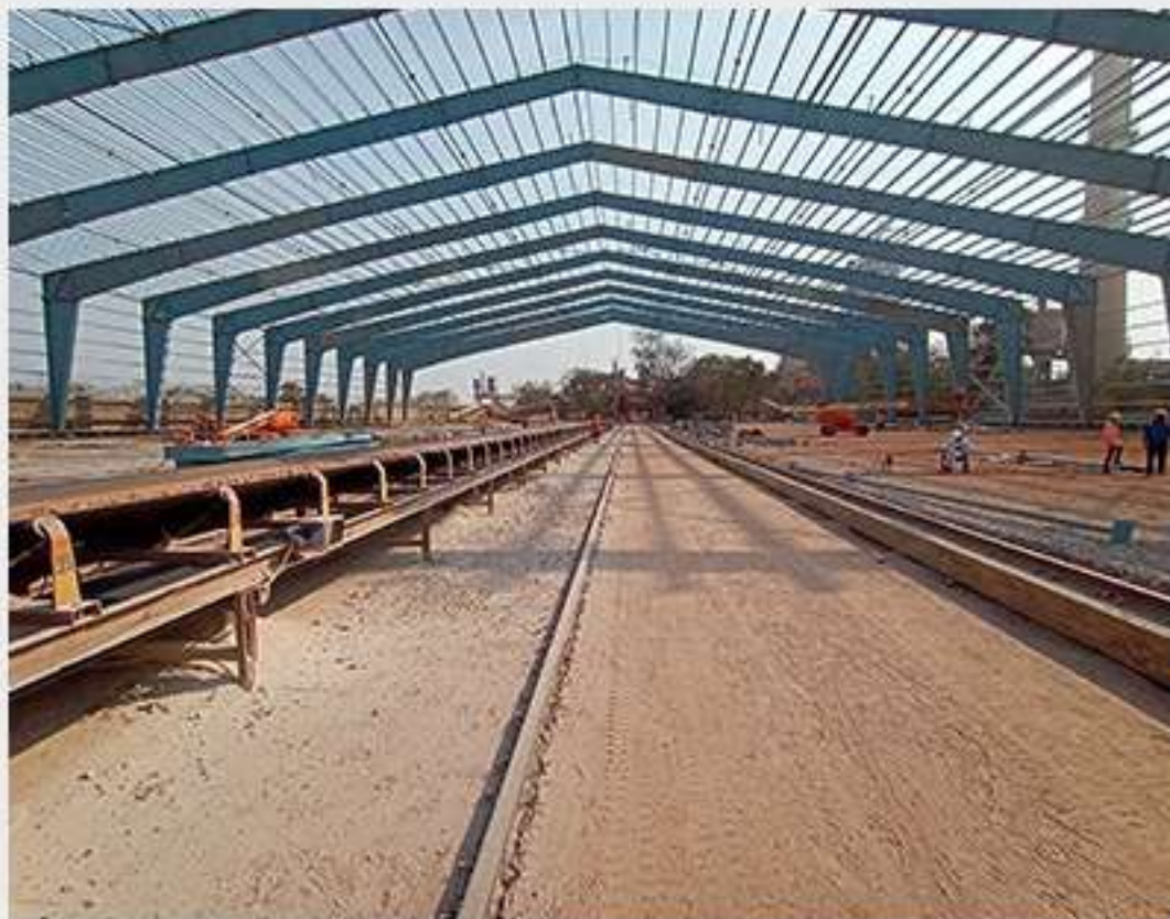
JK CEMENT LTD LIME STONE COVERING SHED Nimbahera, Rajasthan Clear Span building of 85 m
