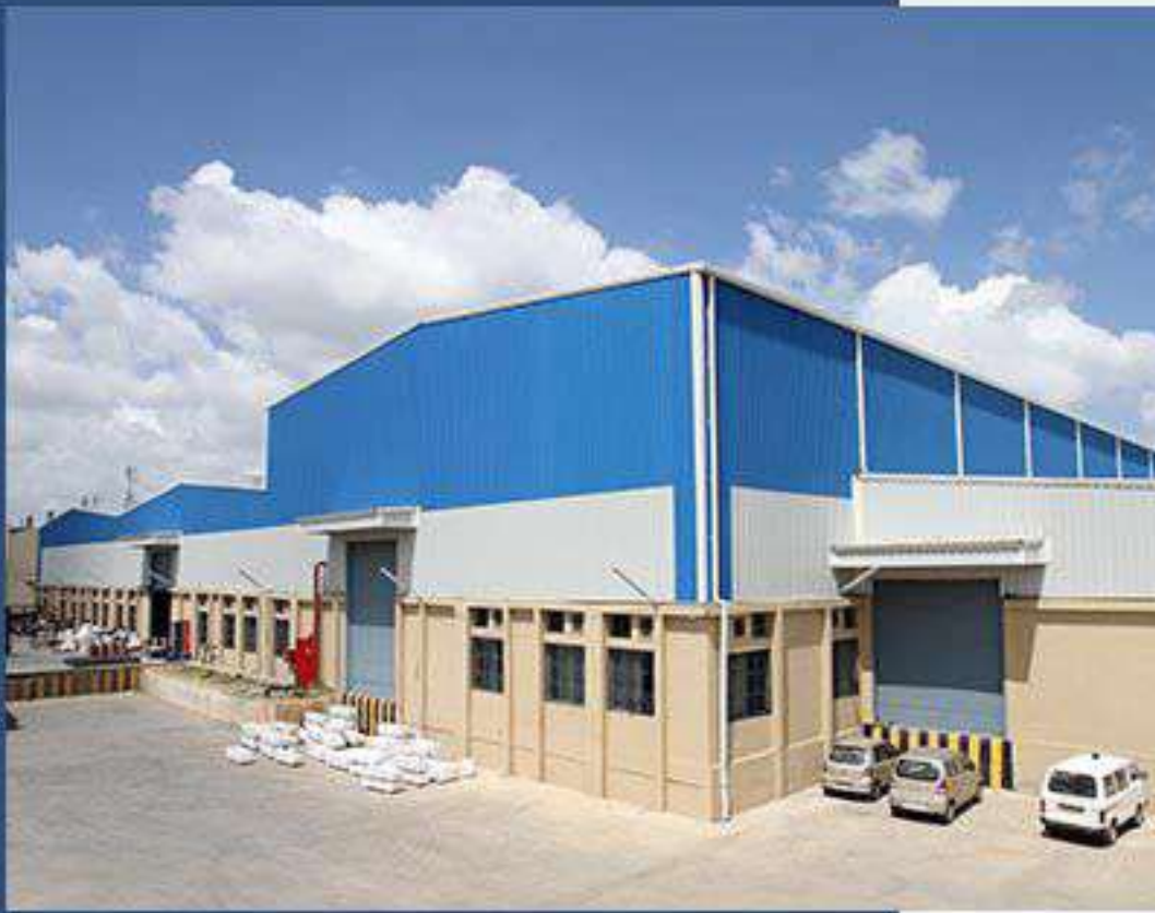
TRACK COMPONENTS PVT LTD GREENFIELD MANUFACTURING UNIT Bangalore, Karnataka
