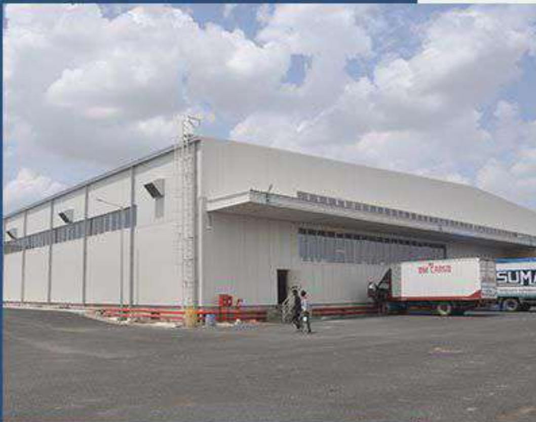
SUBROS LTD GREENFIELD MANUFACTURING UNIT Sanand, Gujarat
