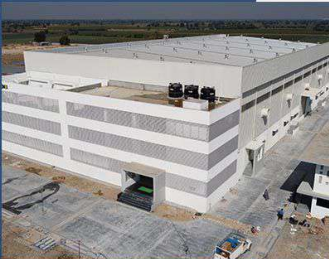
SEKISUI DLJM MOLDING PVT LTD GREENFIELD MANUFACTURING UNIT Mandal, Gujarat
