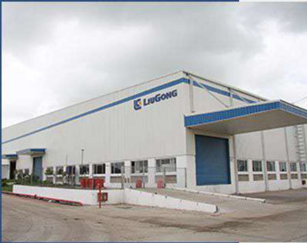
LIUGONG INDIA PVT LTD MANUFACTURING UNIT Pithampur, Madhya Pradesh
