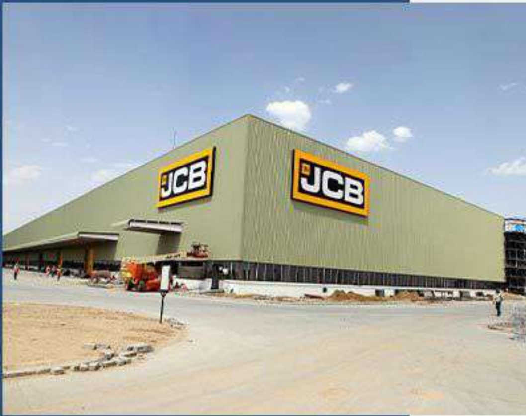
JCB INDIA LTD GREENFIELD MANUFACTURING UNIT Jaipur, Rajasthan
