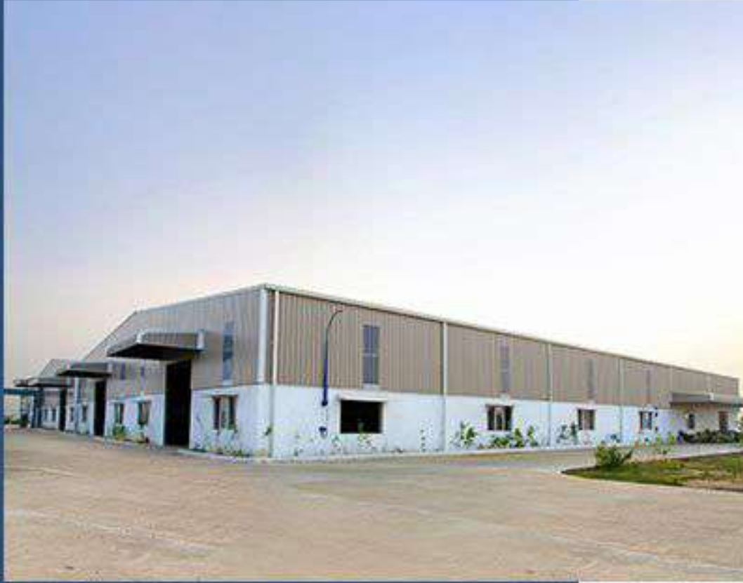
PRABHU LASER COMPONENTS PVT LTD GREENFIELD MANUFACTURING UNIT Chennai, Tamil Nadu
