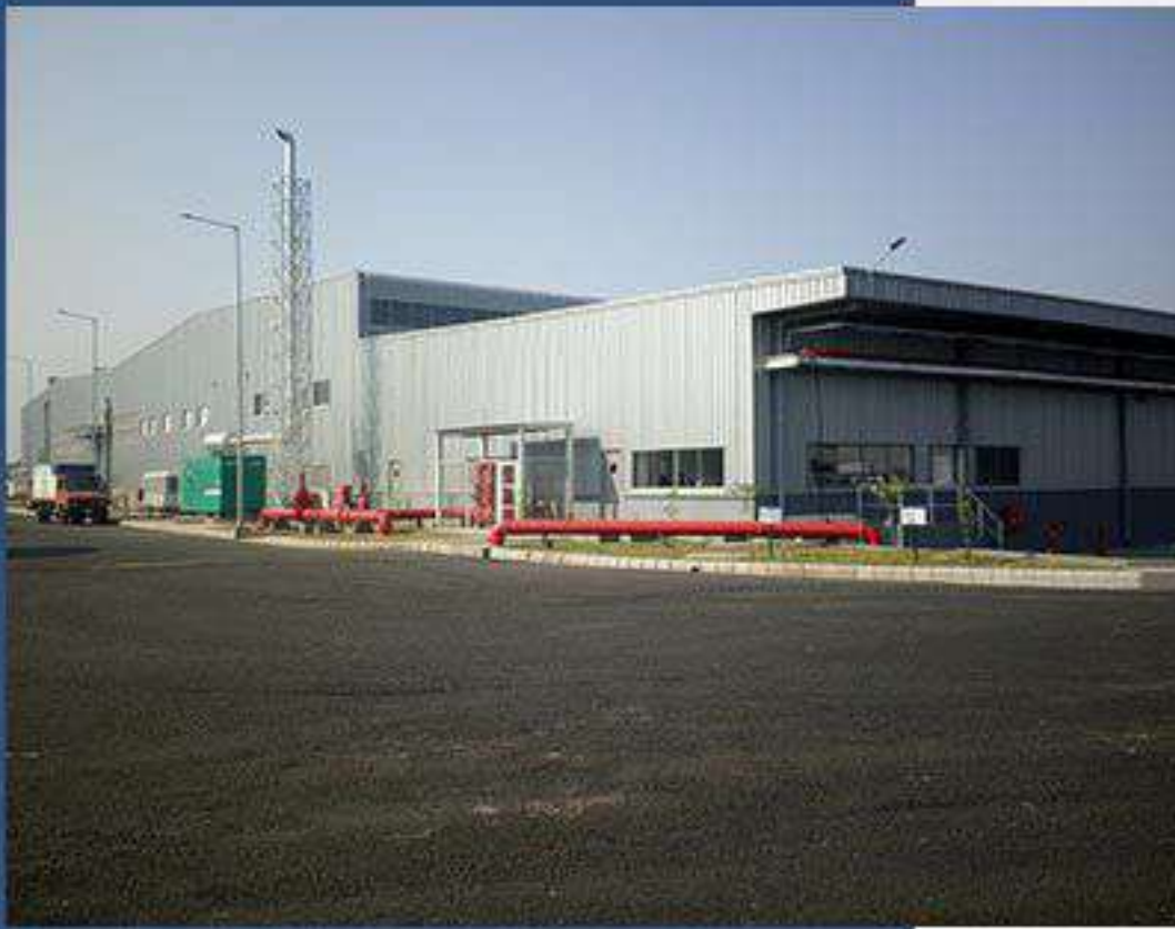
VOLKSWAGEN INDIA PVT LTD CLC WAREHOUSE Pune, Maharashtra
