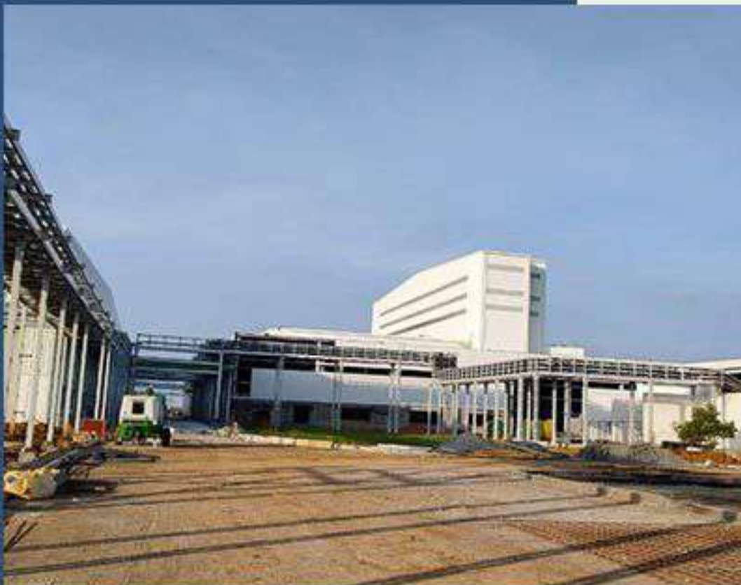
CEAT LTD GREENFIELD TYRE MANUFACTURING UNIT Chennai, Tamil Nadu
