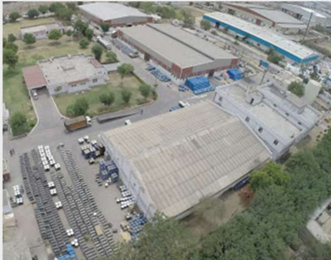
S-CCI INDIA PVT LTD MANUFACTURING UNIT Bhiwadi, Rajasthan
