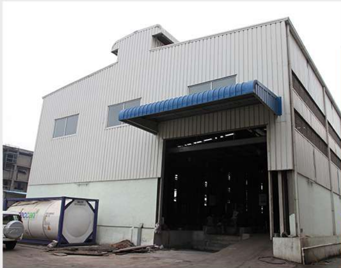
ANUPAM RASAYAN INDIA LTD WAREHOUSE Surat, Gujarat
