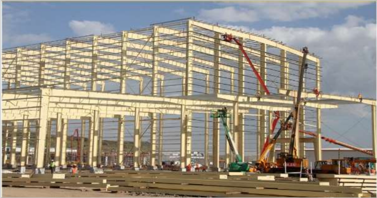
(b) Secondary framing systems
