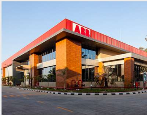
ABB INDIA LTD GREENFIELD MANUFACTURING UNIT Nashik, Maharashtra
