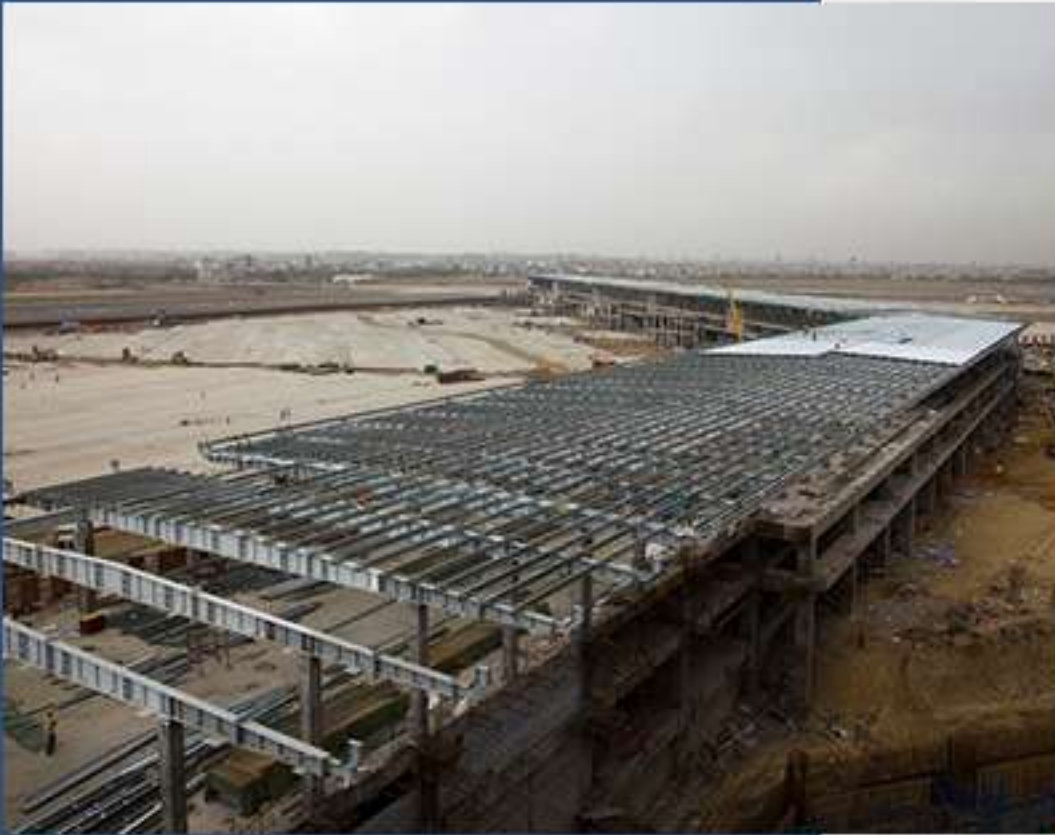
DELHI INTERNATIONAL AIRPORT LTD (AIRPORT AUTHORITY OF INDIA) AIRPORT TERMINAL (7 LAYERED ROOFING SYSTEM) New Delhi
