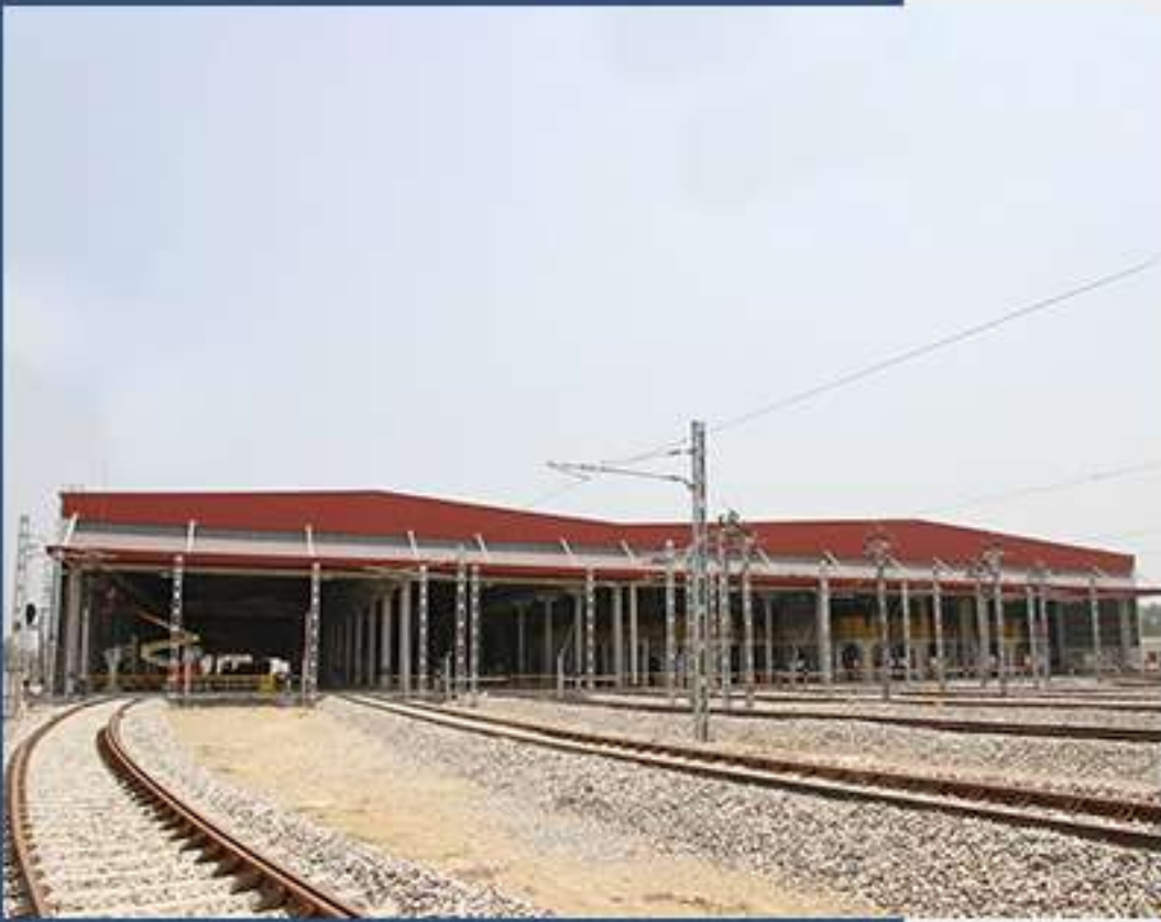
MADHEPURA ELECTRIC LOCOMOTIVE PVT LTD (INDIAN RAILWAYS) MAINTENANCE DEPOT Saharanpur, U.P.
