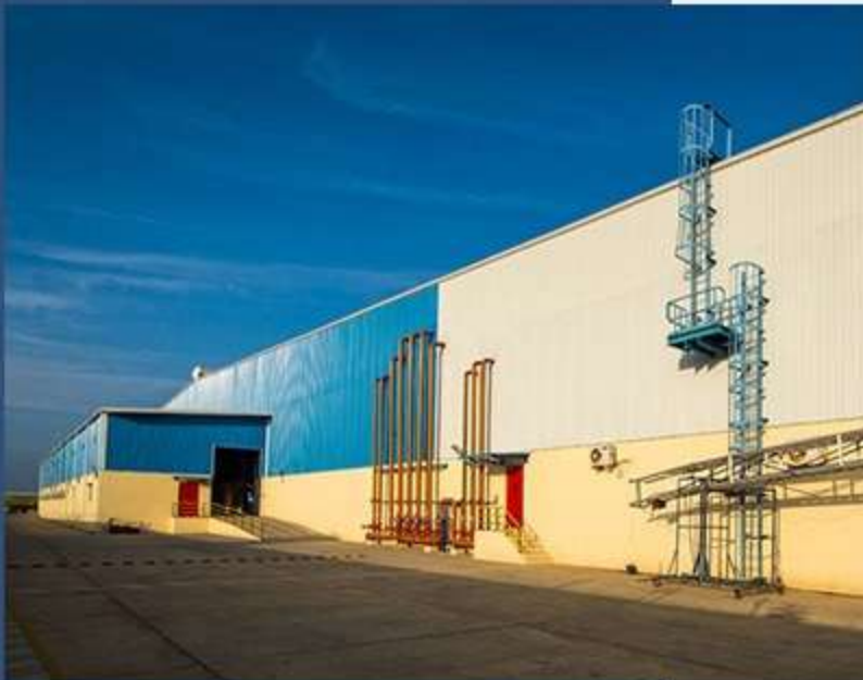
POLYTRUSIONS INFRASTRUCTURE LLP MODERN WAREHOUSE Tiruvallur, Tamil Nadu
