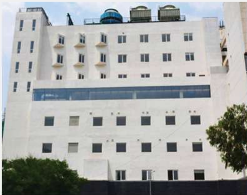
FORTIS HEALTHCARE LTD G+7 HOSPITAL BUILDING Bangalore, Karnataka
