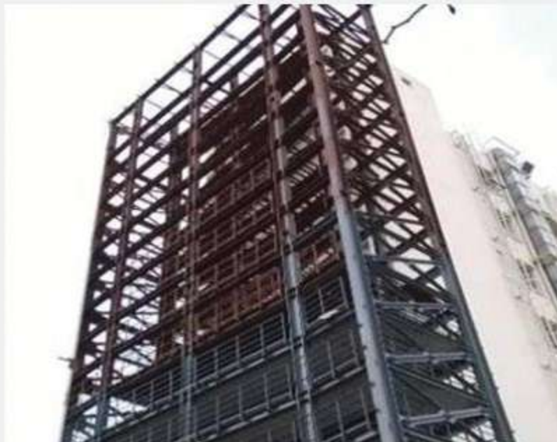
FORTIS HEALTHCARE LTD EMERGENCY EXIT RAMP STRUCTURE Chennai, Tamil Nadu
