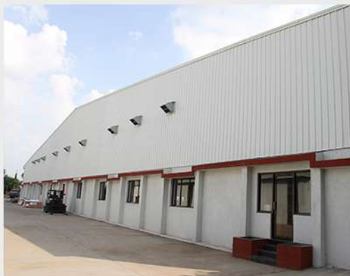
ABB INDIA LTD MANUFACTURING UNIT Vadodara, Gujarat
