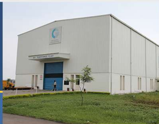
CG POWER AND INDUSTRIAL SOLUTIONS LTD MANUFACTURING UNIT Malanpur, M.P.
