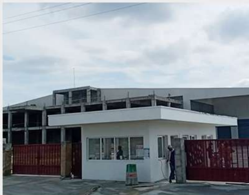
DECCAN ENTERPRISES LTD MANUFACTURING UNIT Sultanpur, Telangana
