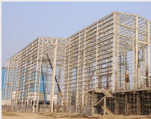
GE T&D INDIA LTD VALVE HALL & GIS BUILDING Kurukshetra, Haryana
