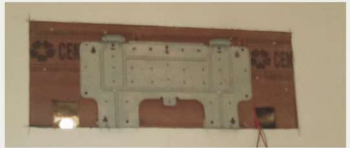
Wall AC Fixing Arrangement
