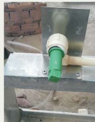
Tap Fixing Arrangement
