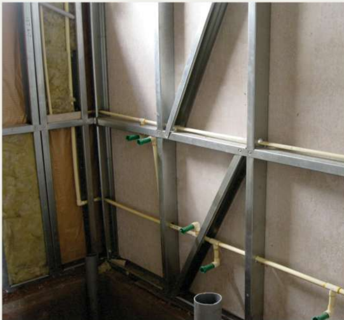
Arrangement of Pipe line for Various Services
