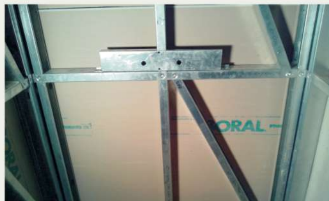
Wash Basin Fixing Arrangement
