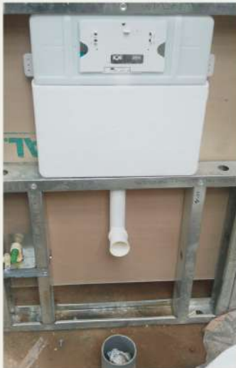
Wall / Floor mount WC Fixing Arrangement
