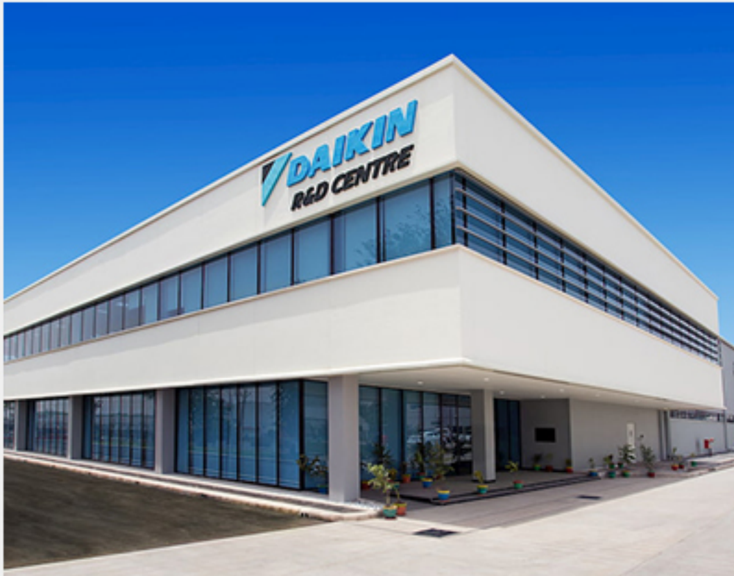
TAKENAKA INDIA PVT LTD (DAIKIN AIRCONDITING) R&D CENTER Neemrana, Rajasthan
