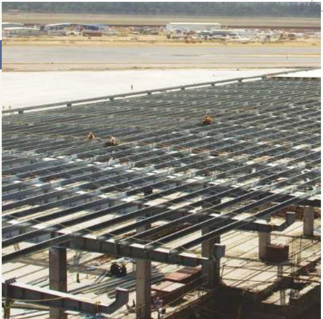
Pre-Engineered Structural Steel Systems - IGI Airport Terminal 3, PERS
