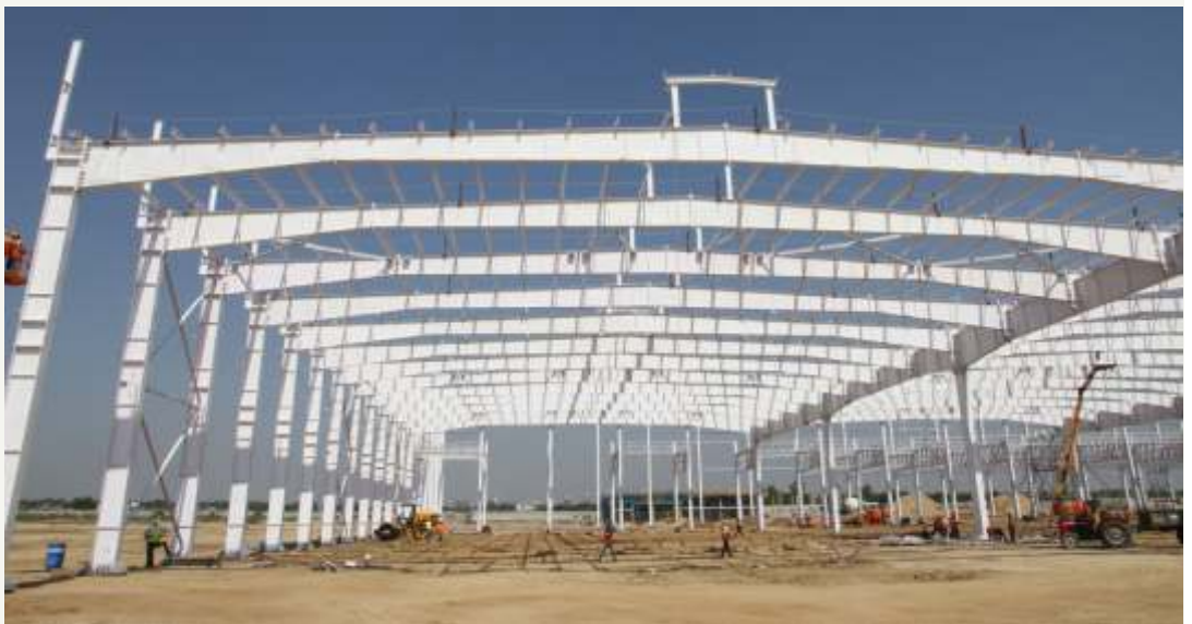
Typical Primary and Secondary Framing Systems
