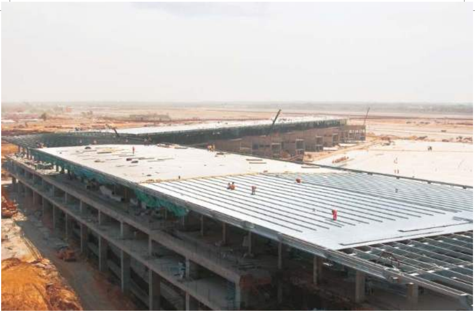
Standing Seam Roofing System - IGI Airport Terminal 3, PIERS
